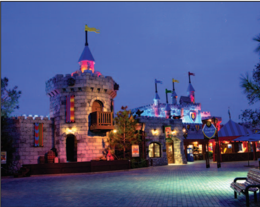
Gallegos Lighting added magic to this Legoland theme park with Permacolor dichroics. Photo by Gallegos Lighting.
